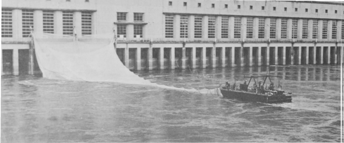
Figure 27.—Giant net strains the entire discharge of a turbine and leads the fish to the barge below Bonneville Dam. Captured fish are observed to see how turbines affect their survival.
