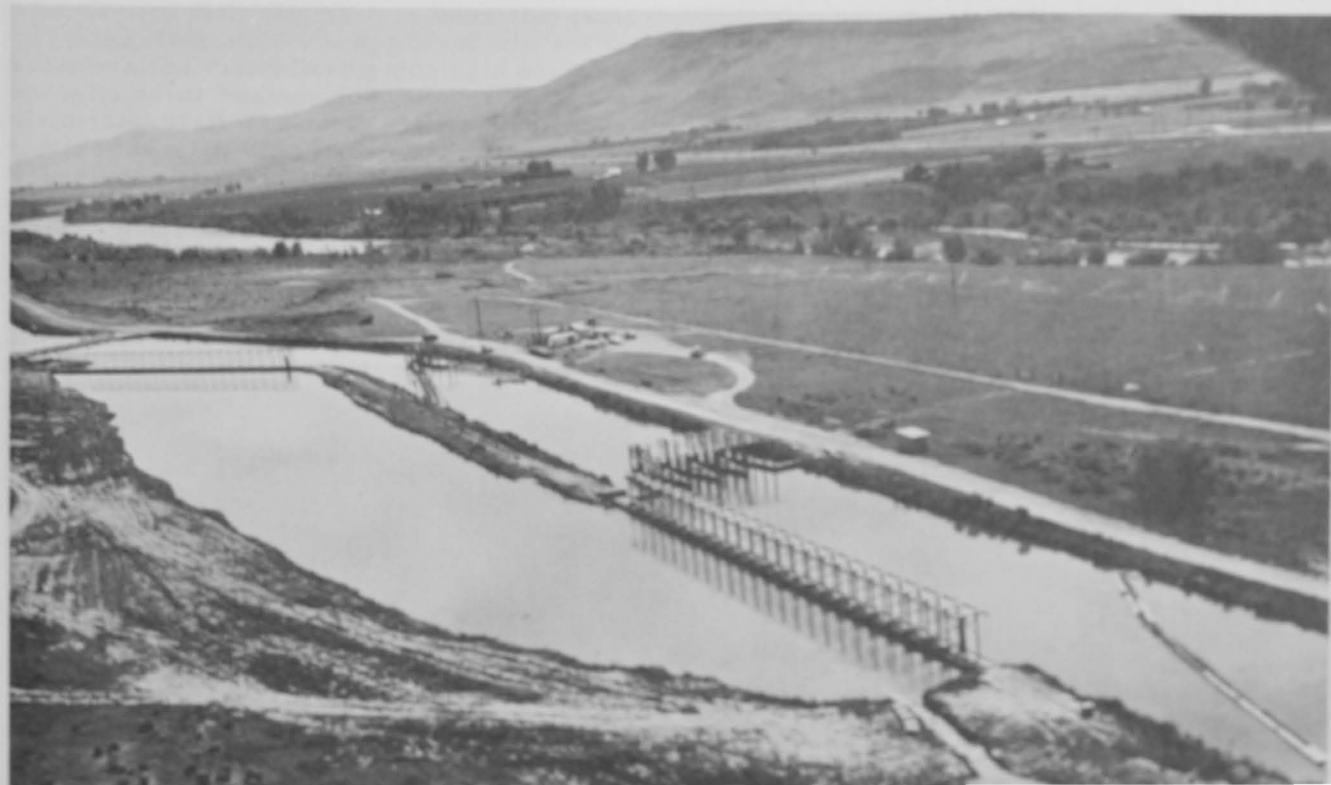
Figure 11.—Prototype of electrical field installation to guide juvenile salmonids.
