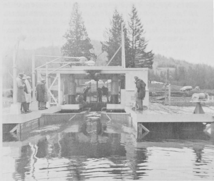
Figure 16.—Experimental artificial floating outlet used in collection experiments at Ariel Dam.
