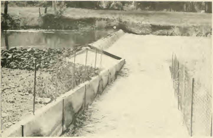
FIGURE 24.—Dam constructed across creek to divert adult salmon up fishway and into holding ponds. (See also fig. 1.)
