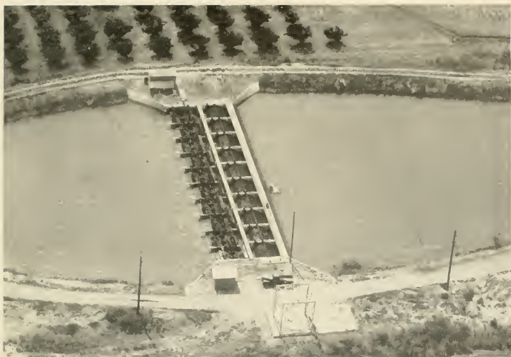
FIGURE 10.—Revolving fish screens in irrigation canal. Waterflow from right to left.
