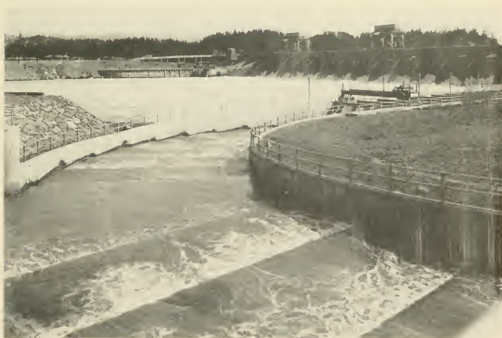
FIGURE 7.—Fishways in foreground and on far shore at Bonneville Dam on the Columbia River.
