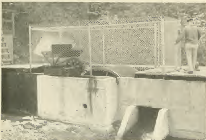
FIGURE 18.—Revolving screen in water supply flume diverts fish and debris back to stream at Little White Salmon Hatchery of the Fish and Wildlife Service.
