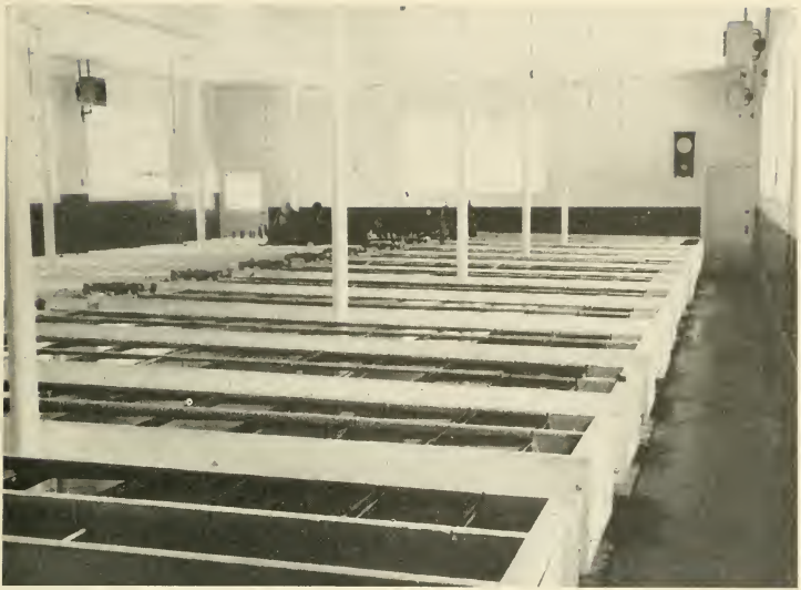
FIGURE 20.—Interior view of Quilcene, Wash., Hatchery of the Fish and Wildlife Service. Double-deep-type troughs contain baskets of salmon eggs.
