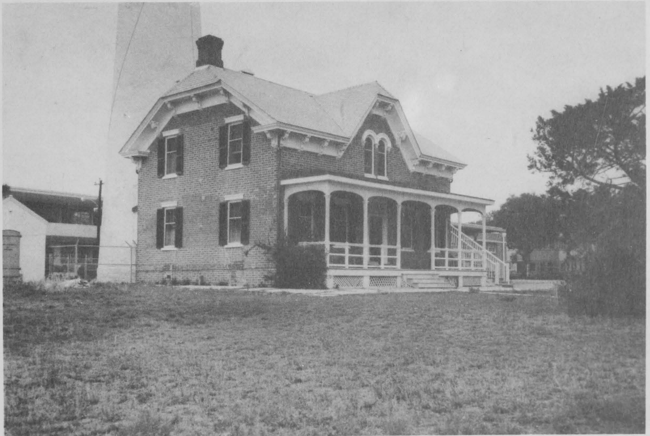
Figure 20.--The former St. Simons Light Attendant Station renovated as an office for the South Atlantic Fisheries Explorations Program.
