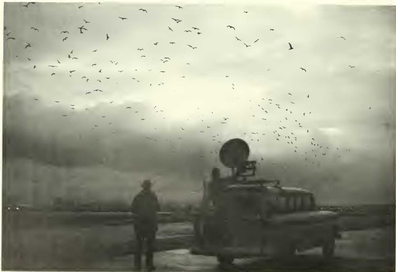
Bird-frightening devices, particularly the recorded distress calls of offending species, have been used successfully in driving starlings from city roosts, gulls from airfields, and blackbirds from feedlots. In application, the calls are recorded on tape and later amplified and broadcast from trucks having sound equipment. On disks, the calls can be "broadcast" with ordinary record players. Recording (top), and gulls being dispersed from the Moffett Naval Air Station in California. (Photo by Denver Wildlife Research Center, top; U.S. Navy, bottom)
