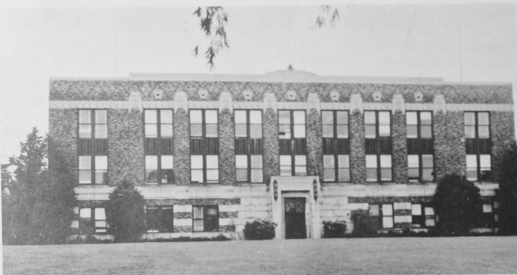
▲ The original "Montlake Laboratory" is now an integral part of the Bureau's research complex. Built in 1931, it housed all the Bureau's research activities until recent years. This now historic building has been the scene of many international commission meetings, where decisions of importance to world fisheries have been made.
