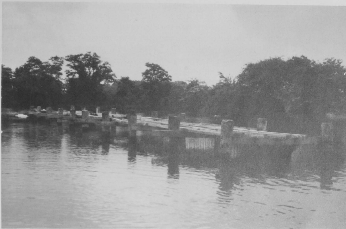
Figure 2. --Wooden structure, 108 x12 feet, capable of supporting 4,000 strings of seed oysters. This framework is located in Boone Creek, a natural salt-water pond adjacent to the laboratory in Oxford.
