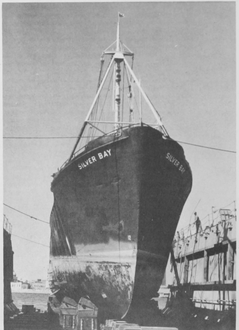
Figure 27.--Shipyard haulout and maintenance are integral parts of the safety program.
