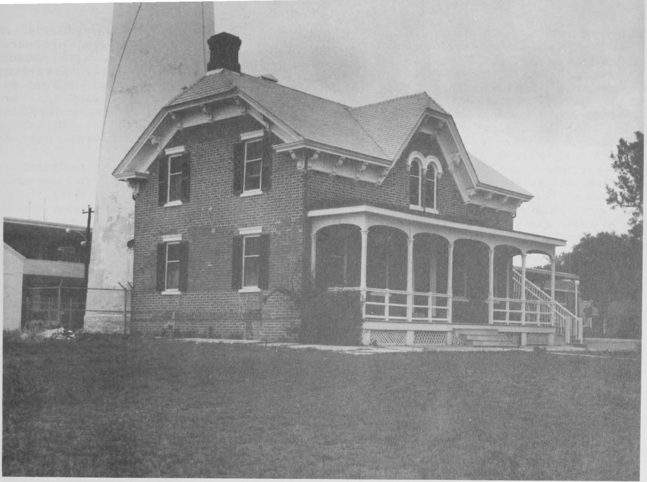
Figure 13.--St. Simon Island Light Attendant Station renovated for office facility.
