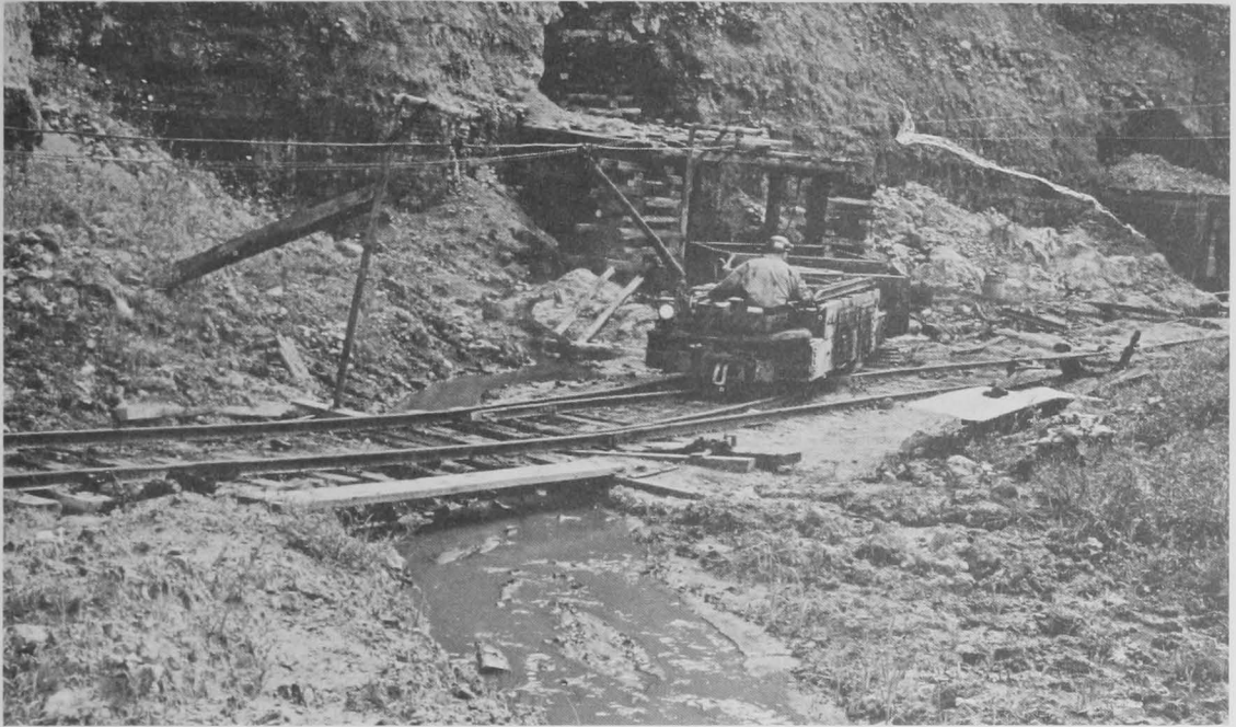
Figure 7. -- Acid discharge from recent coal drift mine opening (pH 2.85).
