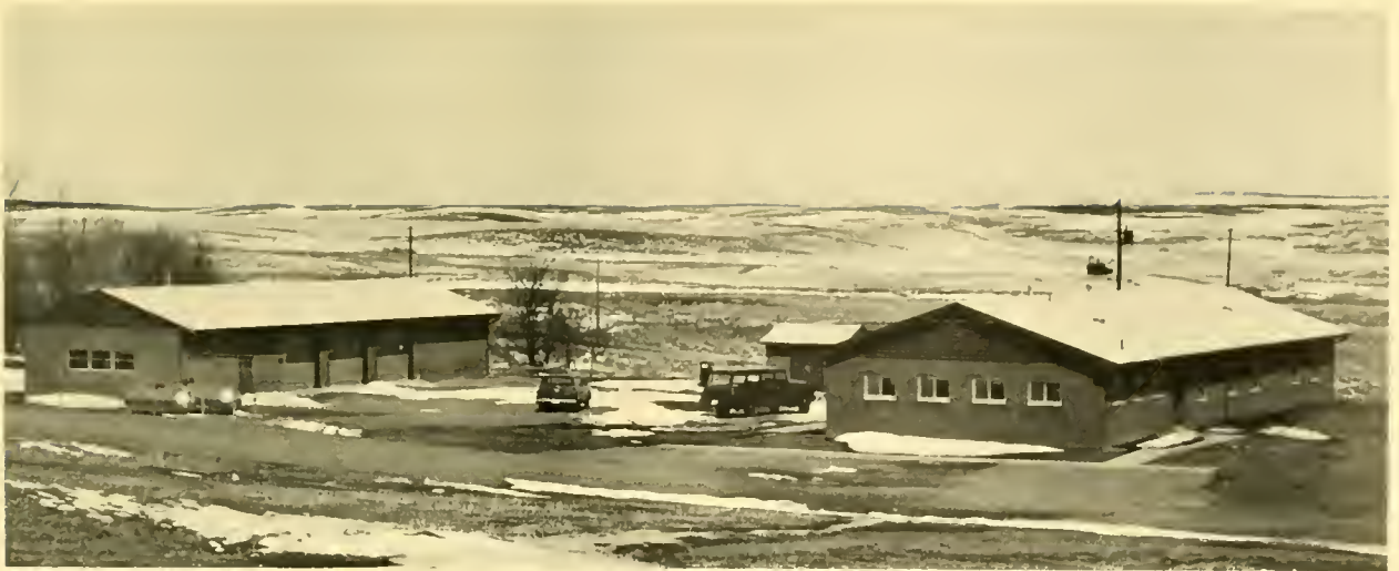
Headquarters of the Woodworth Station of the Northern Prairie Wildlife Research Center near Jamestown, N. Dak. The laboratory is on the right, and the pumphouse and garage-service building are to the left. (Photo by Harvey K. Nelson)
