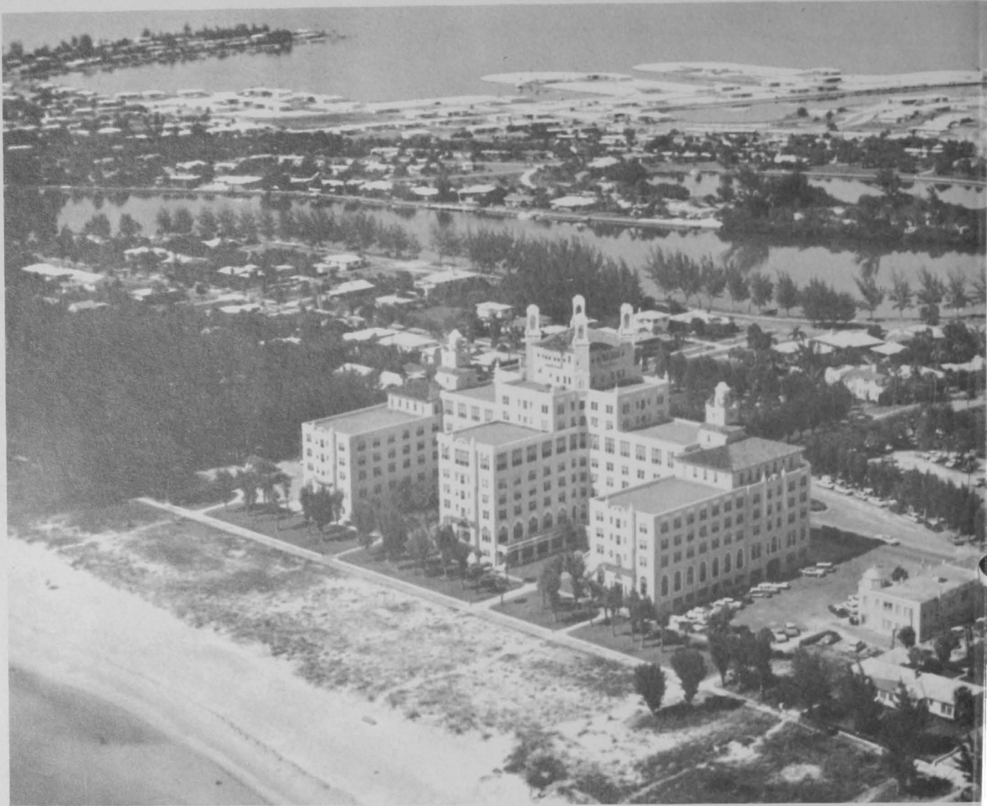
The Regional Office at St. Petersburg Beach occupies the 6th and 7th floors of the Don CeSar Federal Center, a former luxury hotel on the Gulf of Mexico. The building in the lower right corner is the Biological Field Station.
