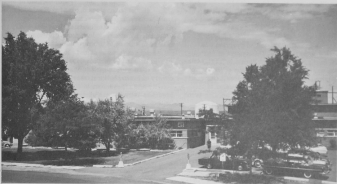
Fish-Pesticide Research Laboratory, Building 45, Denver Federal Center
