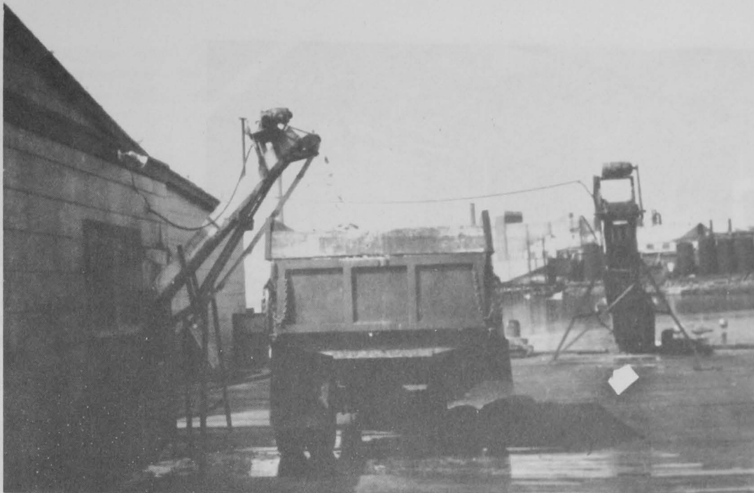
Figure 12.--A conveyor drops the gurry into a truck for shipment to the dehydration plant.
