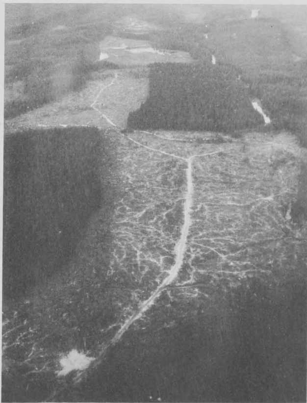
Within the next decade much of Southeastern Alaska's over-age timber will be harvested in logging operations like the one that has been carried on at Katlian Bay the past few years.
