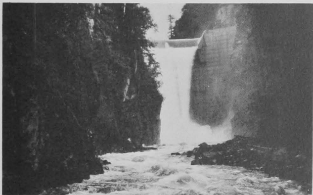
The Blue Lake Dam near Sitka is the forerunner of many large dams that will be constructed on Alaska's lakes and streams.
