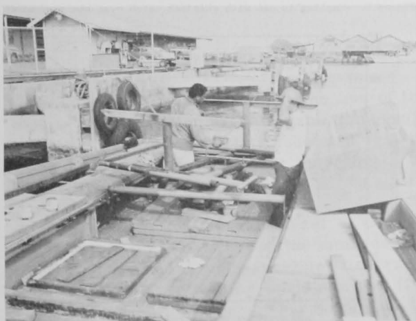
Figure 6a.--Installing framework of the turntable.
