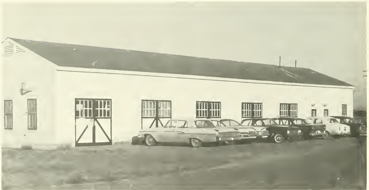
The new nutria research station at Houma, La., which will provide office and laboratory space for research and control biologists assigned to study this pestiferous rodent. (Photo by A. Loren Ward)
