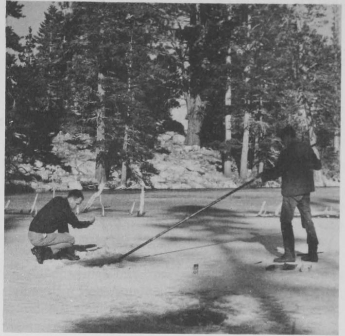
Figure 1:--Core sampling the bottom sediments of a small, ice-covered Sierra Nevada lake.
