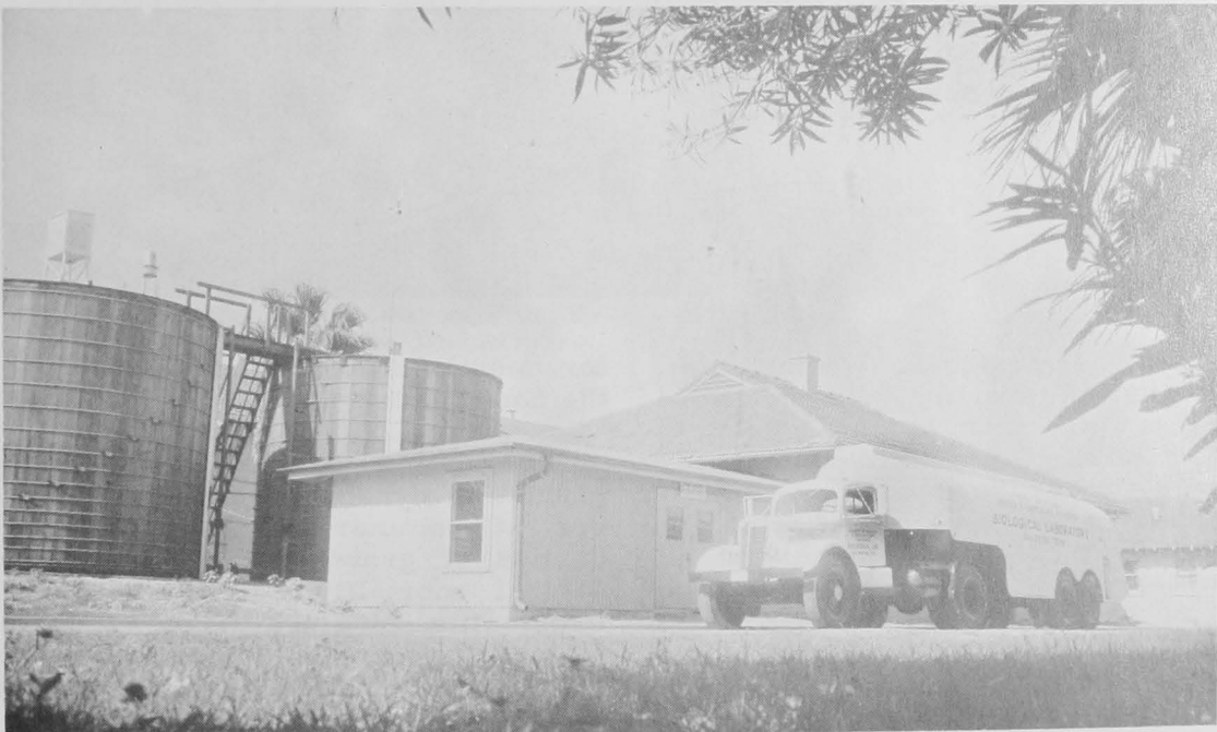
General view of recirculating sea-water system (Building D) showing storage tanks, pump house, and sea-water truck.
