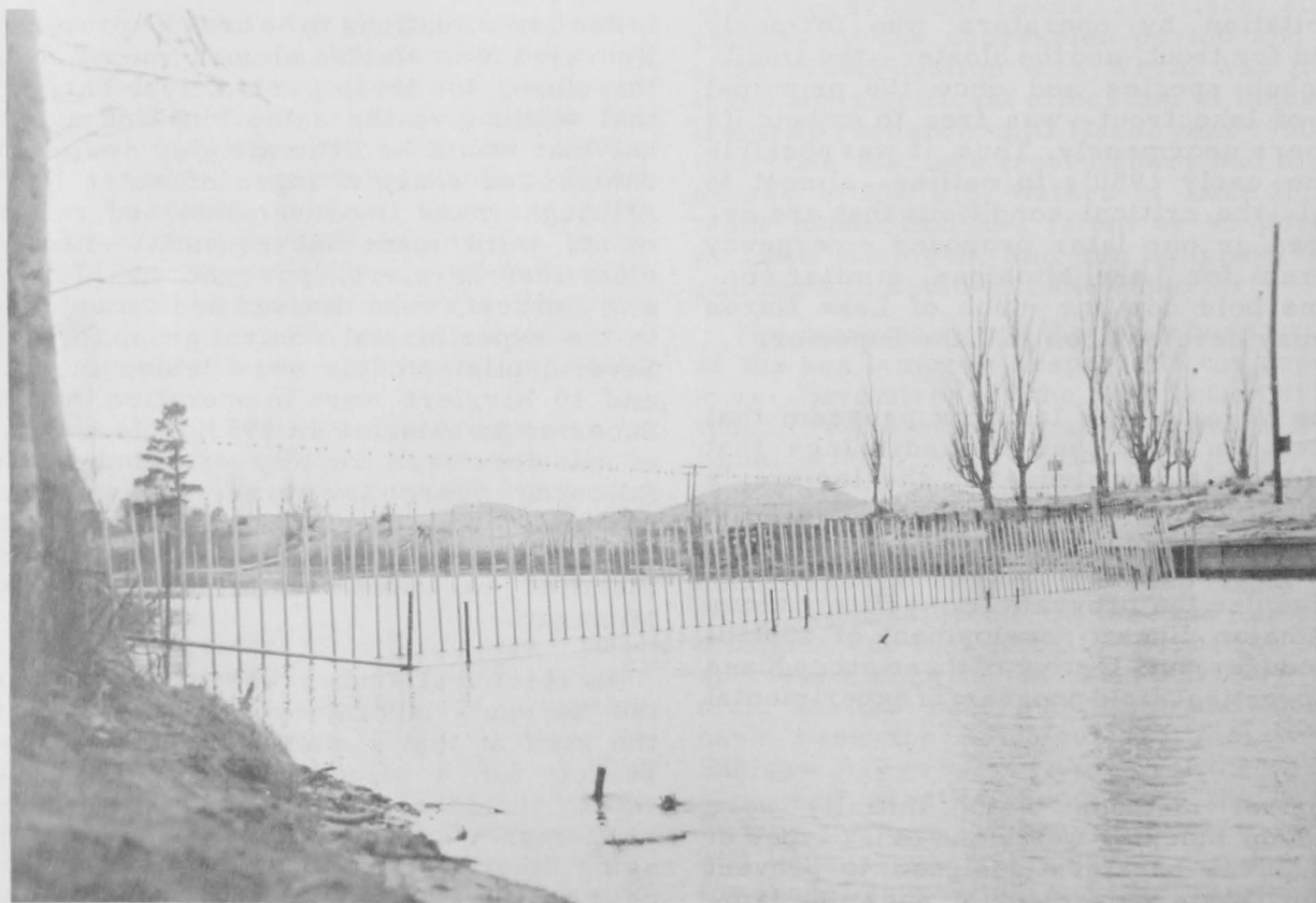
Direct-current barrier used to block sea lamprey spawning runs at Two Hearted River, May 1957.
