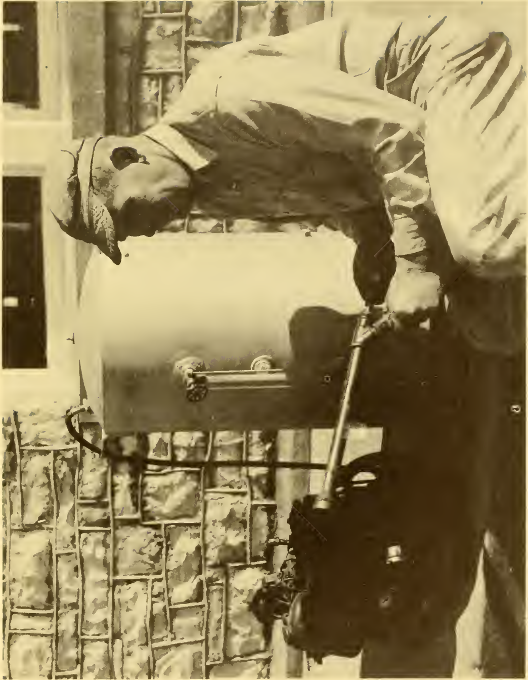
Figure 7.--Gun-type tree sprayer, air compressor and pneumatic tank used in weed control operations.
