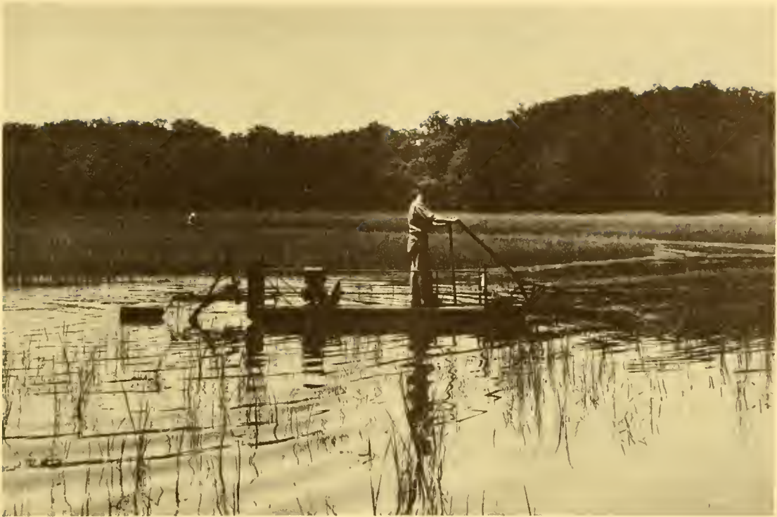
Figure 5.--Hockney underwater weed cutter (courtesy George C. Hockney)!
