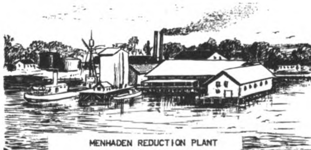
MENHADEN REDUCTION PLANT
