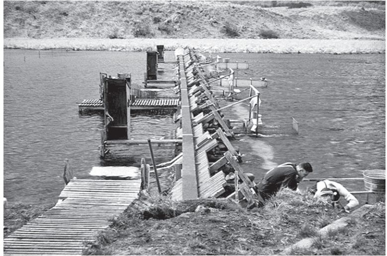
Karluk River weir (center), counting huts (left), and smolt traps (right), 1957. (Robert F. Raleigh, Saint George, UT)
