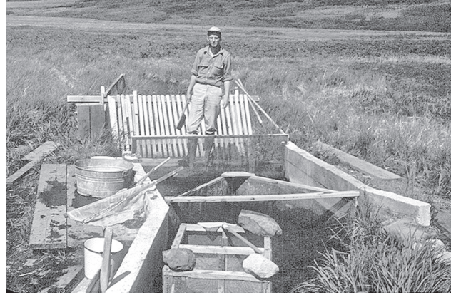
Bare Lake outlet, weir, and salmon research gear, 1954. (Clark S. Thompson, Shelton, WA)
