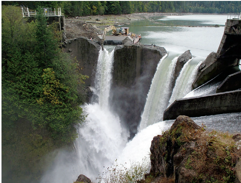
The Glines Canyon Dam, in Washington State, in the early stages of being dismantled.
