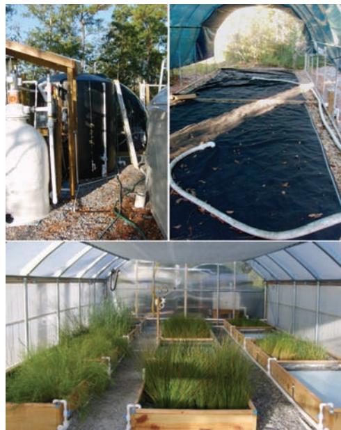
Figure 8. Multitrophic Reclamation System used to reclaim high nitrogen, high sediment wastewater. Upper left is the bead filter for initial particle removal followed by geobag in upper right for fine particle entrapment. The water then flows through seagrasses in the greenhouse for nitrogen removal (lower picture).
