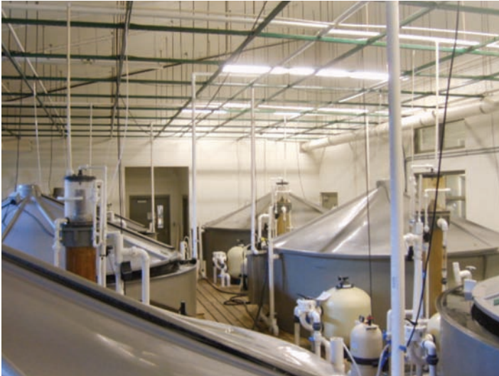
Figure 2. Aquaculture Visitors' Pavilion Broodstock Tanks. The broodstock tanks all have temperature and photoperiod control as well as closed, recirculating filter systems.
