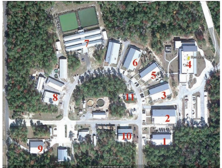
Figure 1. Aerial view of the Thad Cochran Marine Aquaculture Center site at Cedar Point. (1) Red Snapper Broodstock and Larval Rearing Building, (2) Aquaculture Visitors' Pavilion, (3) Aquaculture Growout Building, (4) Research Building, (5) Aquaculture Demonstration Laboratory, (6) Red Snapper Growout Building, (7) Shrimp Production Greenhouse, (8) Shrimp Maturation and Hatchery Buildings, (9) Fish Health Building, (10) Wet Laboratory Building and (11) Multi-Trophic Reclamation System.
